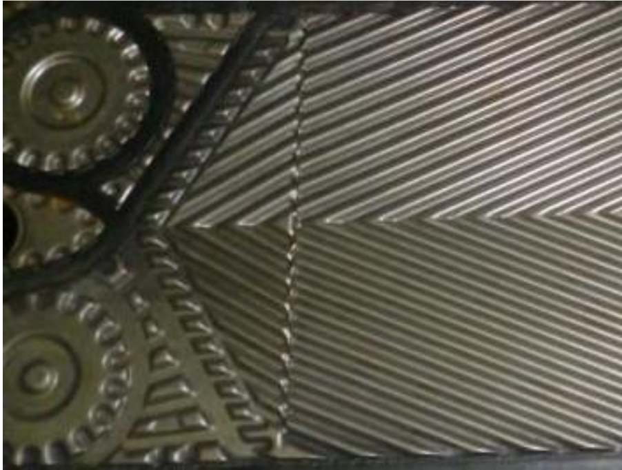
Fresh Water Generator protected with HASYTEC DBP after 6 months
